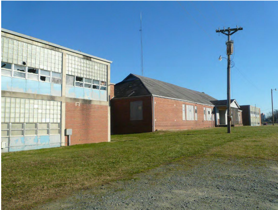
Figure 1: Historic 1937 building in center
