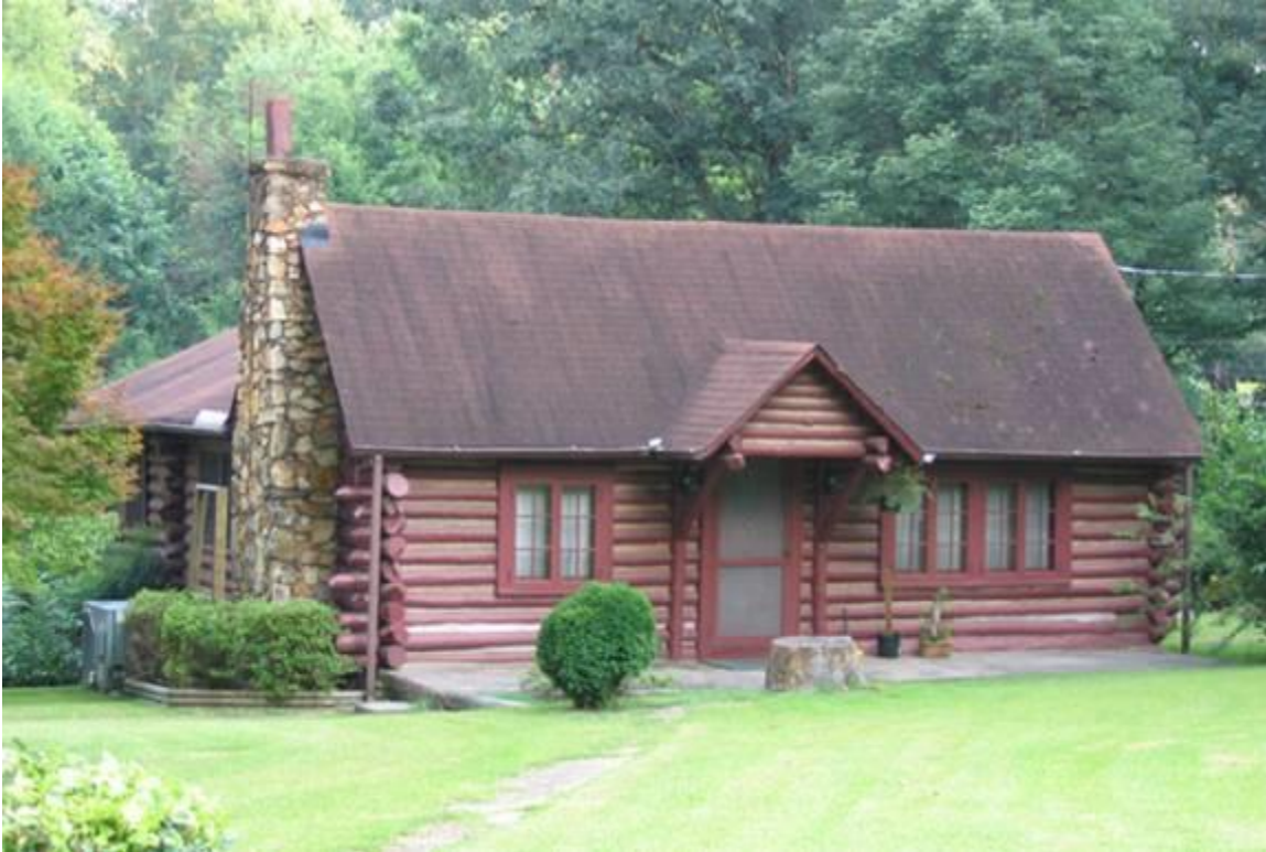
Bobby McConnell House, ca. 1940 6216 Hunter Avenue, Derita
