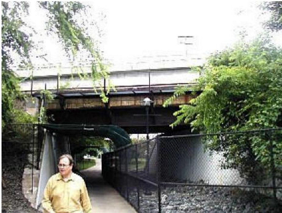
Piedmont and Northern Railroad Trestle Charlotte, N.C.
