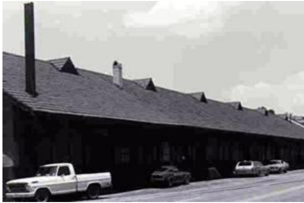
Piedmont and Northern Freight Depot, Charlotte, N.C. (Destroyed)
