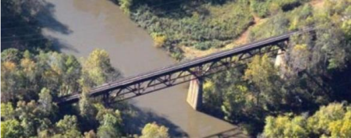
Piedmont and Northern Railroad Bridge over South Fork River, Gaston County
