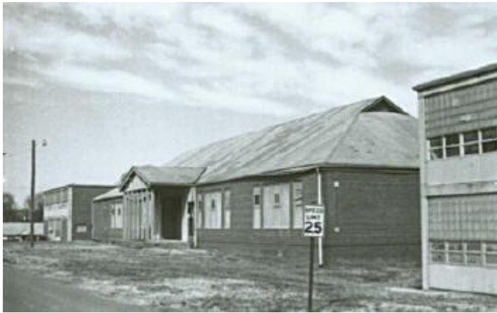
19. Torrence-Lytle School 1937 302 Holbrooks Rd.
